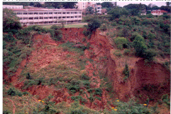
F. Threats of destruction of a College following crumbling
