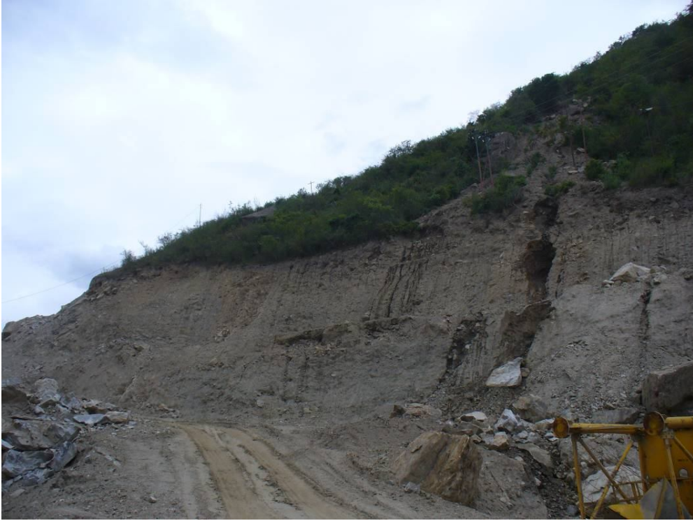
Punatsangchhu Dam site under construction
