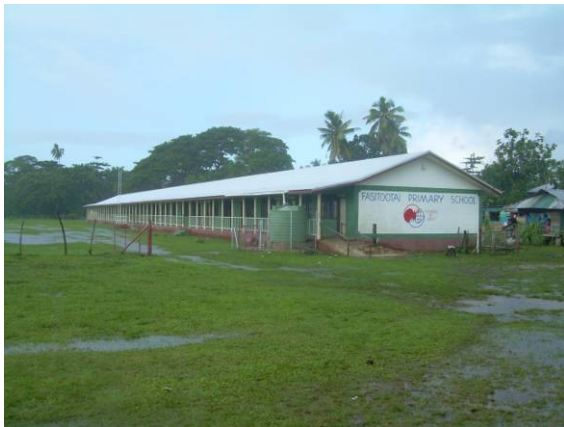
Fig. 25 Village primary school within Project Site
