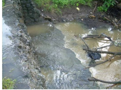
Fig. 6. Drain discharge into mangroves
