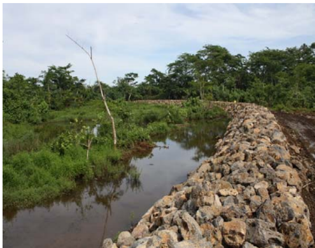
A retaining stone wall to protect the coastal ecosystems from flooding
