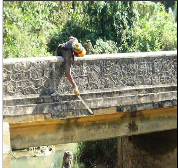
A farmer points out the usual high-water mark during flooding episodes. More intense flooding is a serious threat to key pieces of local infrastructure, such as this bridge, and could prevent farmers and workers from reaching their fields and jobs, disrupting local livelihoods.
