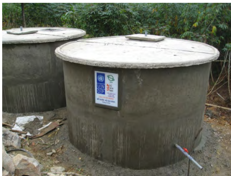
CBA/VN/SPA/08/003 (Cam Tam, Thanh Hoa) Rainwater Harvesting – the new technology introduced in the project area
