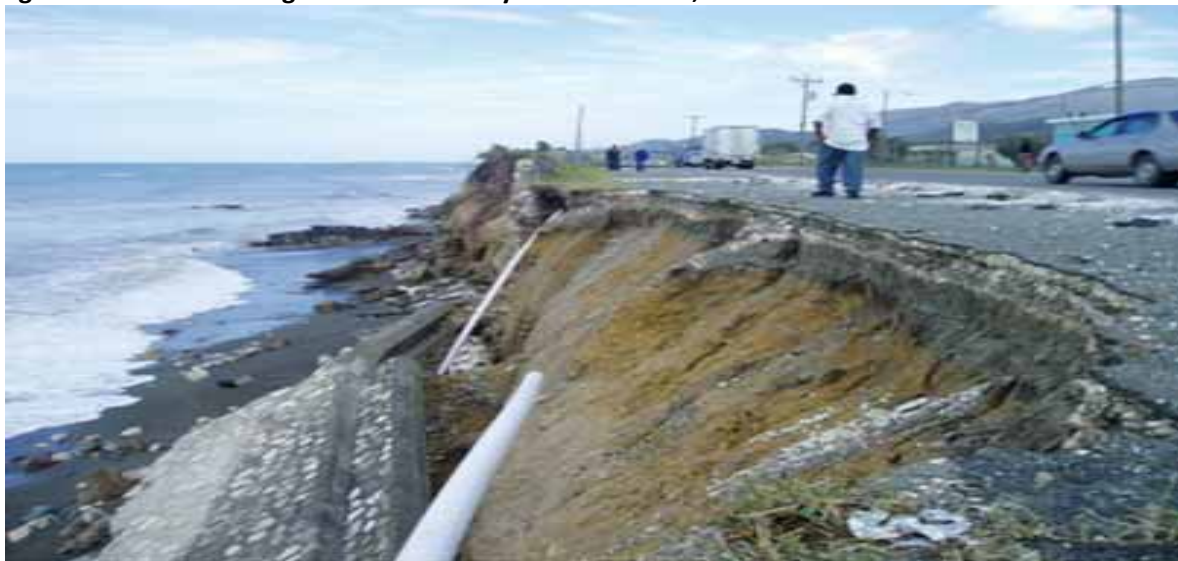
Figure 4.27: Medium High Cliff Cut in Easily Erodible Marls, Southeast Coast of Jamaica
