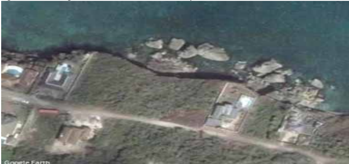
Figure 4.28: Housing on Cliff above Extensive Cliff Collapse, North Coast of Jamaica
