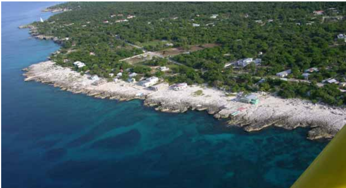
Figure 4.36: Southwest Coast, East of Negril Lighthouse (upper left), showing fractured rocky platform zone without vegetation that is frequently swept by storm waves. Crowded boulders visible at right mark the front of the debris ridge, extending behind the green house
