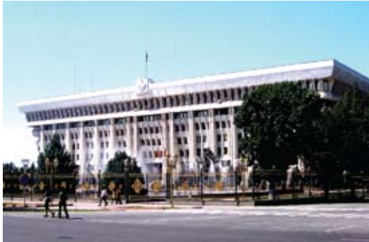
Building of the Kyrgyz Republic Government. Project archive.
