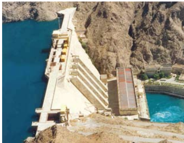
Reservoir is full. Electrical Station Ltd archive
