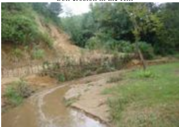
Canal Developed by flowing water from Hill
