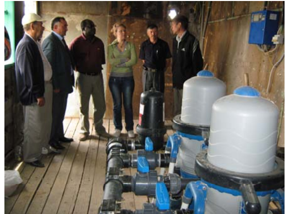
Drip irrigation system installation on the project territory
