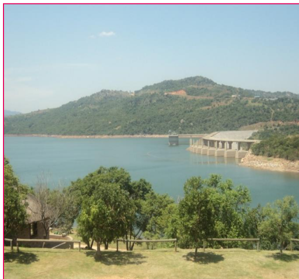
Figure 4.6: A portion of Maguga dam, one of the dams constructed as an adaptation measure in the water resource sector.
