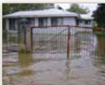
Photo 2: Flooding of residential from heavy rainfall, 2009, SNC Project, MECC, Tonga.
