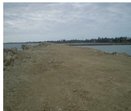
New structures built in 2008 beside Vuna wharf, Nukualofa.
