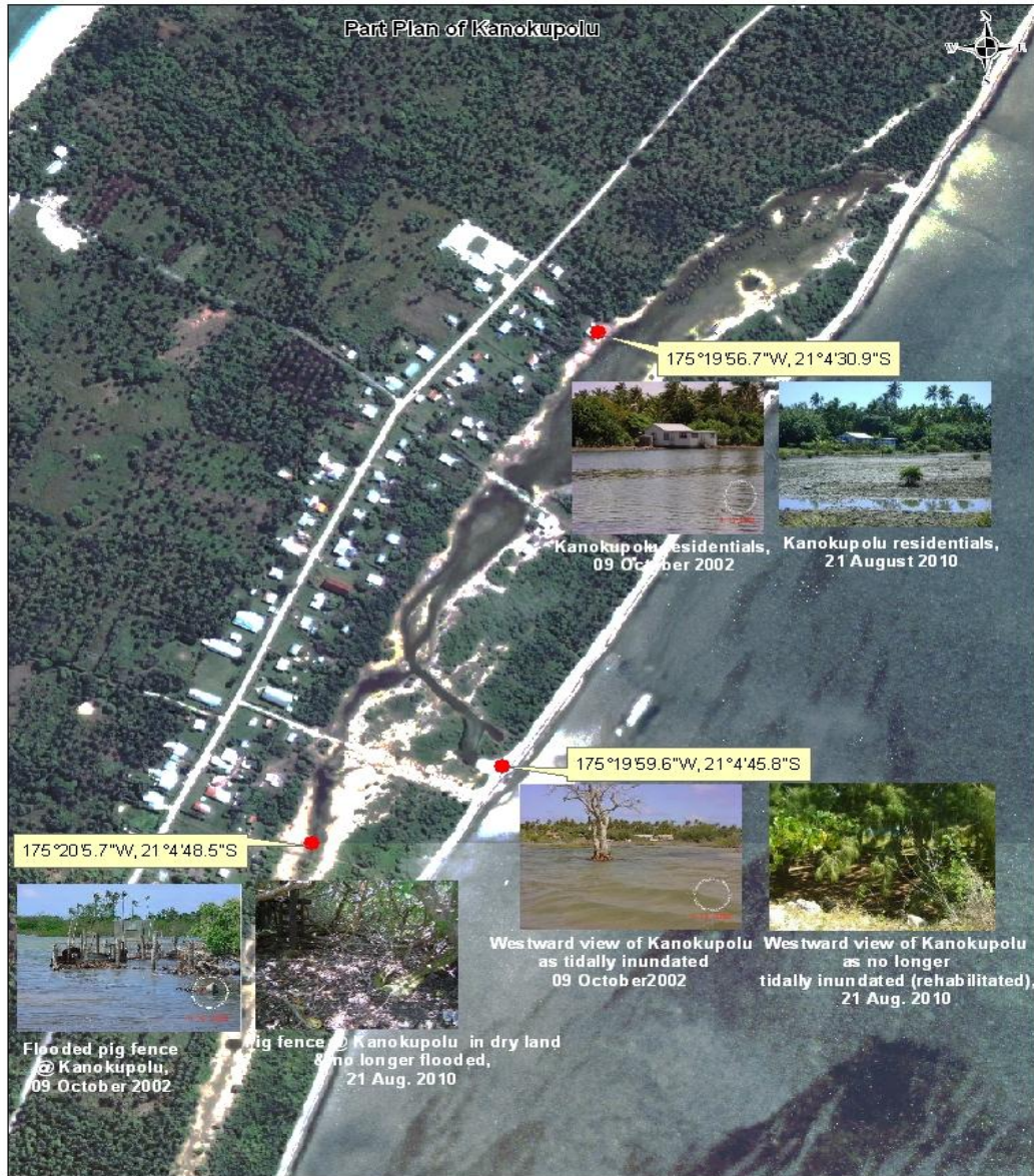
Figure 4.37: Areas in Kanokupolu village that were tidally inundated and also eroded in 2002 (Tonga's Initial National Communication Report). Pictures of these areas were taken in 2010. These areas were rehabilitated after the seawall was completely built in 2005.
