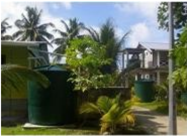
Newly installed household water tanks and guttering to capture and store rainwater. Photo: Jasmine Subasat
