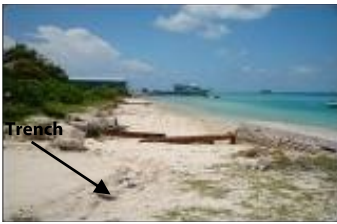
Trench to drain water during flooding on the island of G. Dh. Thinadhoo Photo: ICCRIP project document
