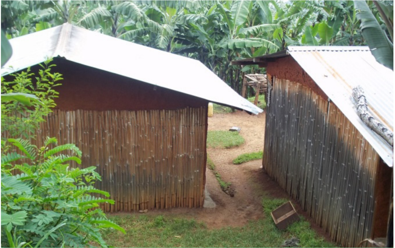
Plate 3.4. Bamboo obtained from Mt. Elgon National Park can be used for protecting house walls from being washed by rain
