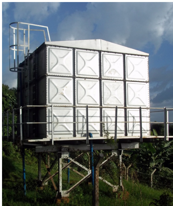
Plate 6.1. An example of a very active and functioning gravity flow scheme at Sipi, Kapchorwa district.
