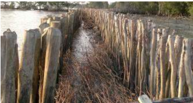
Figure 9(a). Wave break fence
