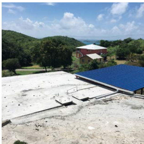
A refurbished water tank on the Grenadine island of Mayreau
