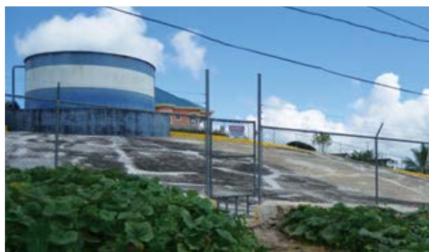
The refurbished ‘barbeque’ water tank in Clarendon, Jamaica
