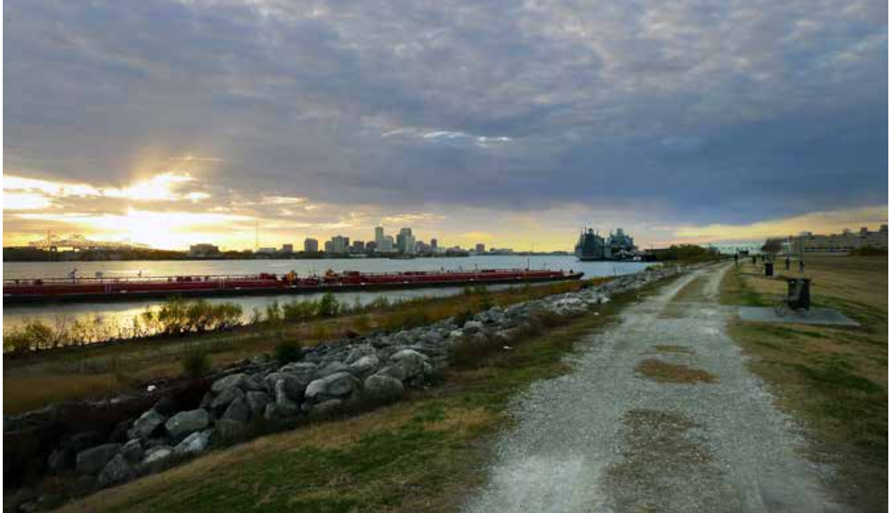
The levee in New Orleans: Lower Ninth Ward © Flickr/Stephen Kennedy
